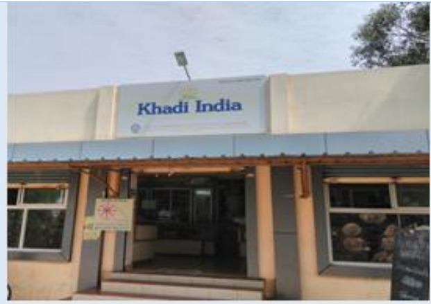
Renovated Sales Outlet
